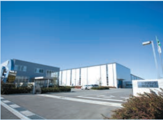
Main plant entrance and office
