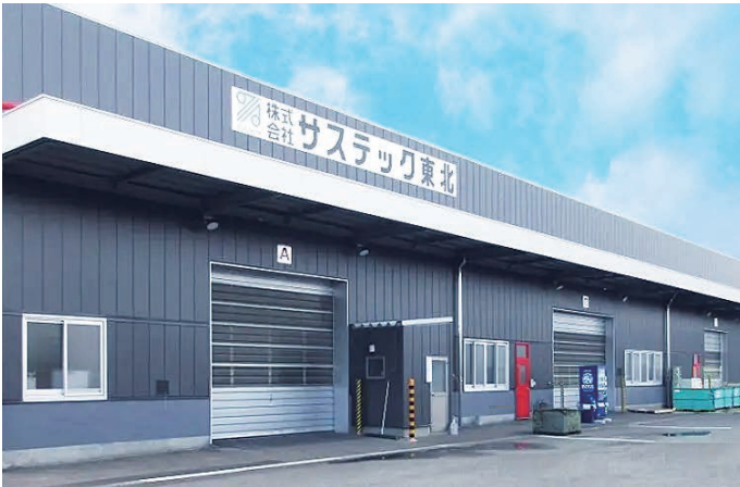
Sus-Tech Tohoku Headquarters Plant facilities overview
