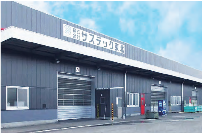
Sus-Tech Tohoku Headquarters Plant facilities overview
