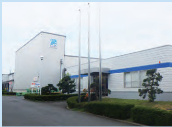
Office and plant building
